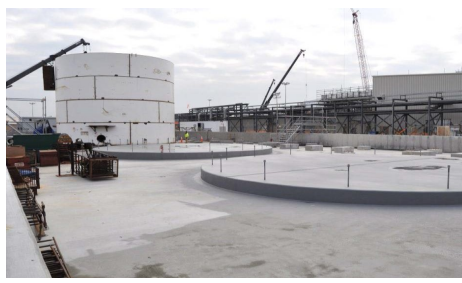
The hydrolysate holding tanks in the hydrolysate storage area (HSA) hold neutralized agent pending lab approval for release to SCWO processing.
