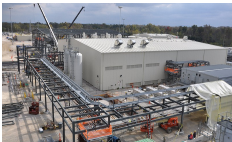
The utility building supplies operating necessities such as steam, air, water, and nitrogen to the facility.
