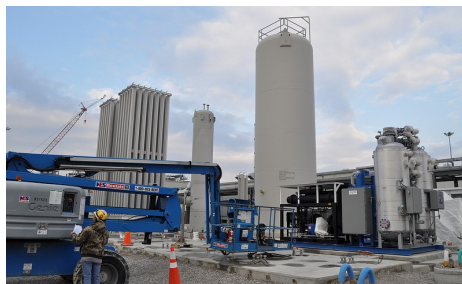
The nitrogen generation plant of the utility building ensures a combustion free atmosphere in the munitions demilitarization building.
